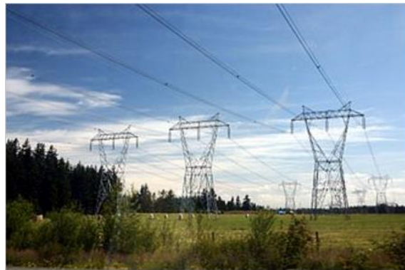
Three-phase electric power transmission lines
